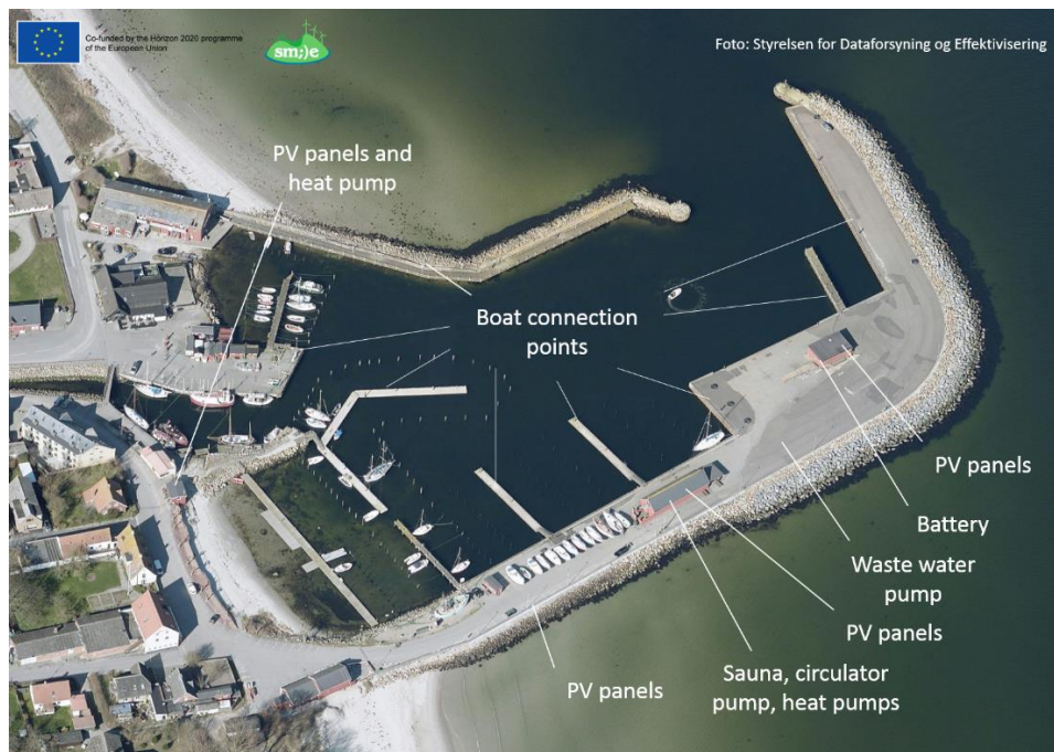
Figure 1. Overview of the Ballen marina with its smart energy components.
