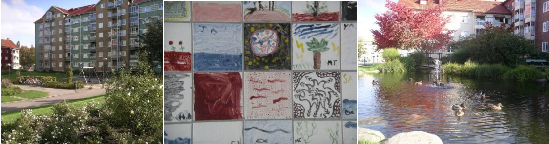
Augustenborg Left: External cladding, new balconies and play spaces, Centre: Public Art and Right: Water attenuation creating pleasant spaces and biodiversity.
