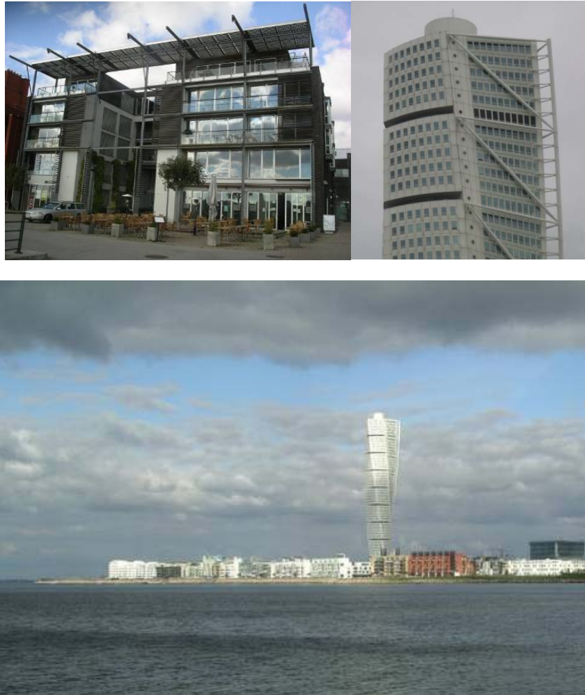
Left: Solar PV array offers some shading to the top flats of this building, Centre and Right: The ‘Turning Torso’, 50 storey landmark of the Western Harbour development
