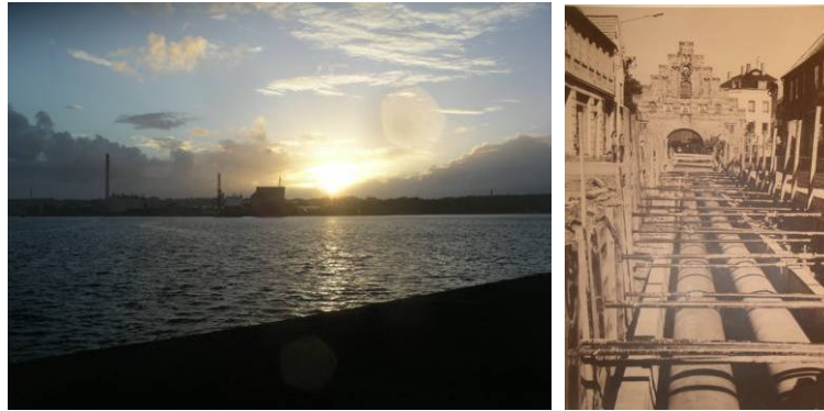
Left: Flensburg power station with its 180m high flue, Right: old photo of original heat mains - ten different ages of heat main now make up the system
