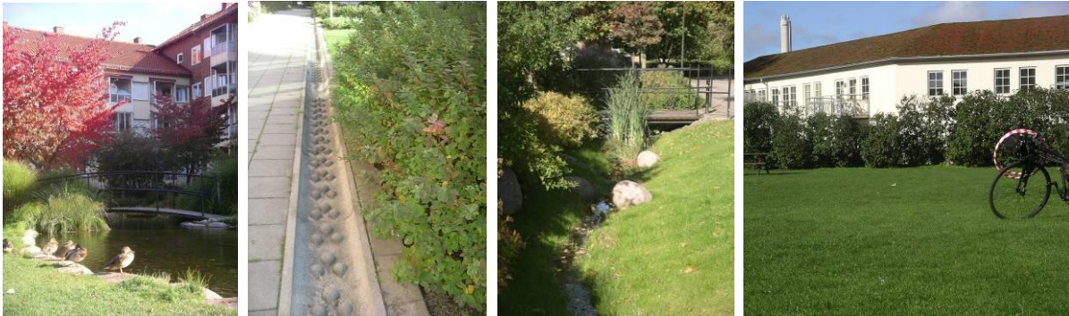
Stormwater control, Augustenborg Left to Right: Attenuation pond, gully, swale and green roof
