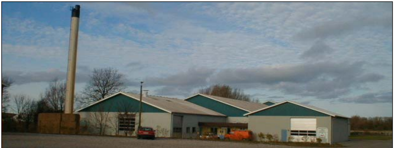
Tranebjerg Heating Plant
