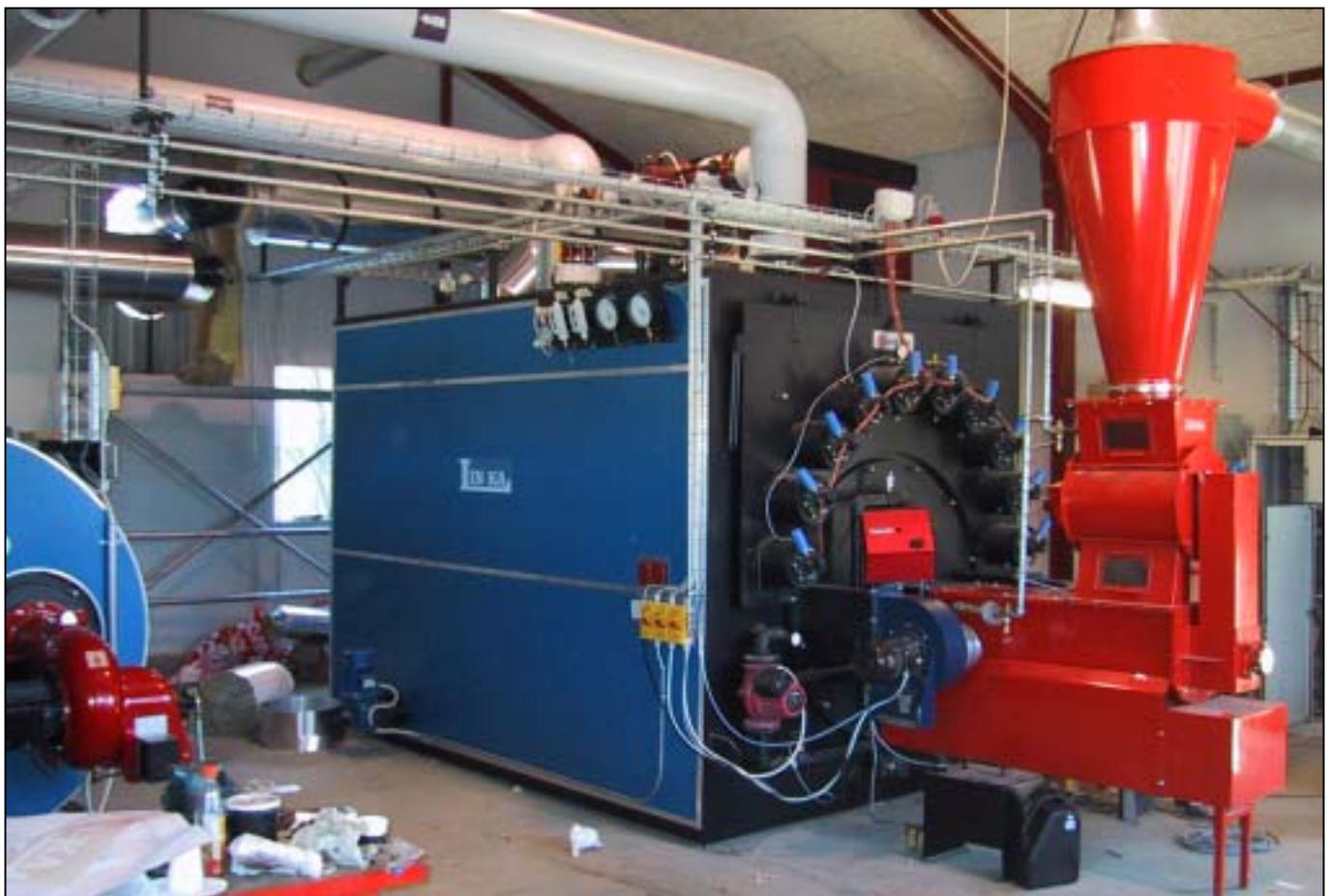
The 800 kW straw boiler at Onsbjerg
