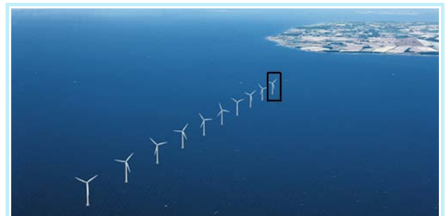
Fig. 1. The partnership Paludans Flak I/S owns wind turbine T1 (framed, Bonus/Siemens 2.3 MW). Picture by Sweco, who did the environmental assessment.
