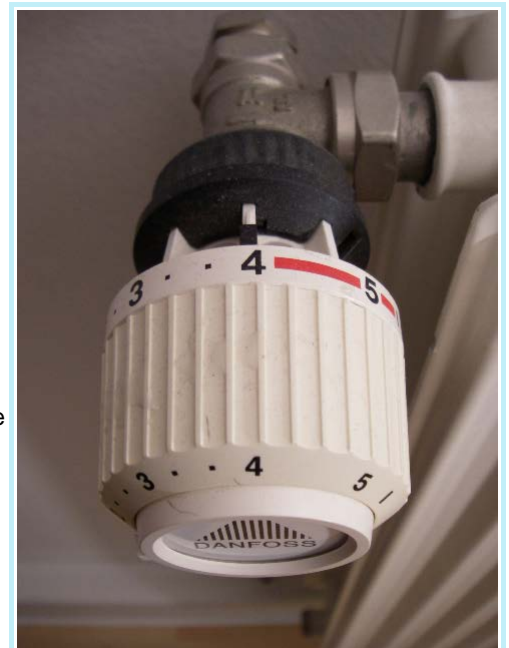
Fig. 1 Thermostat for radiator (Danfoss). Bathroom setting 4 (23 C), living-room setting 3 (20 C), bedroom setting 2 (17 C), staircase and hallway setting (13 C), and anti-freeze setting * (7 C).
