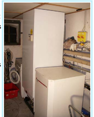
Fig. 1. Heat pump (Klimasol). The smaller box is the heat pump and the tall box contains a hot water storage tank.
