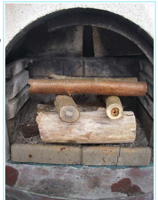
Fig. 1 Supplementary heat. The output depends on fuel weight, moisture, and boiler efficiency rate.
