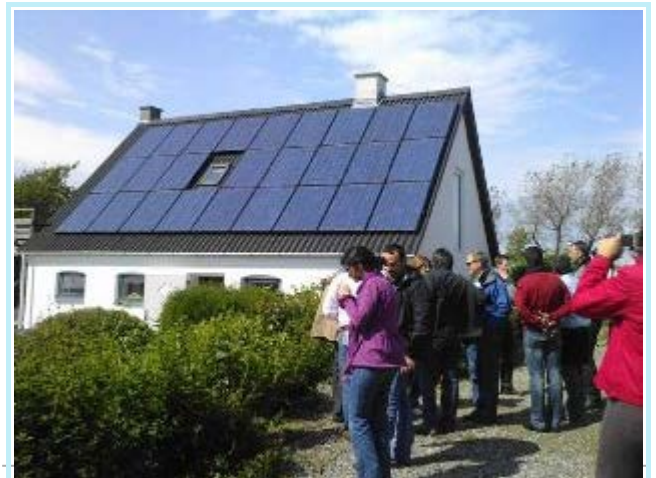
Fig. 1. Photovoltaic panels for a household (Scheuten 5.07 kW, 39 square metres).
