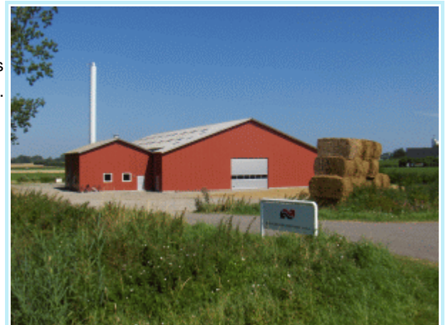
Fig. 1 Ballen-Brundby District Heating Plant
