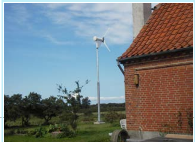
Fig. 1. Household wind turbine (Proven 6 kW). Photo by AB Albrechtsen.
