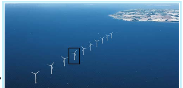
Fig. 1. The partnership I/S Difko Samsø 1 owns wind turbine T7 (framed, Bonus/Siemens 2.3 MW). Picture by Sweco, who did the environmental assessment.
