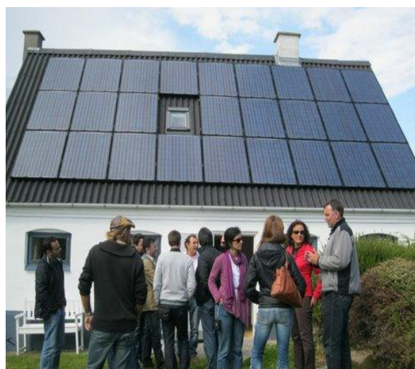
Figure 2. The PV panels cover 39 square meters of the roof.
