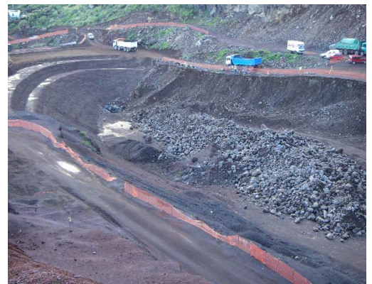
Figure 2. Construction site of the lower reservoir.
