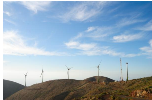
Figure 3. Wind farm, construction site.
