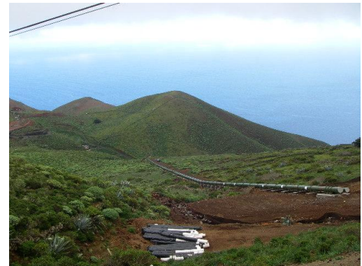
Figure 3. Pipeline to connect the upper and lower reservoirs with a vertical drop of 655 metres.
