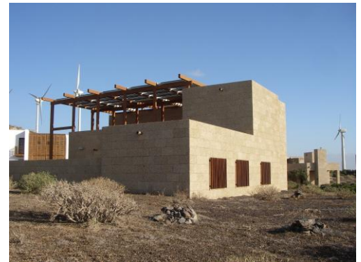
Figure 3. Bioclimatic house (La Tea) in ITER near the Sur airport.
