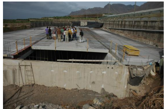
Figure 4. Visit to Biodigester Installation at a Chicken Farm.
