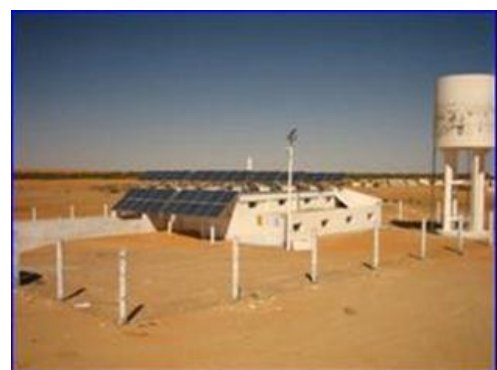
Figure 5. Desalination plant in Tunisia working with PV system
