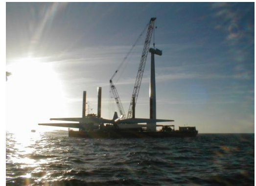
Figure 3. From the construction of 10 wind turbines south of Samsø.
