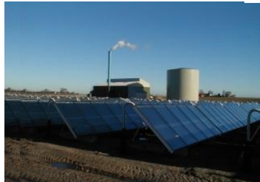
Figure 1. The Nordby-Maarup district heating plant.
